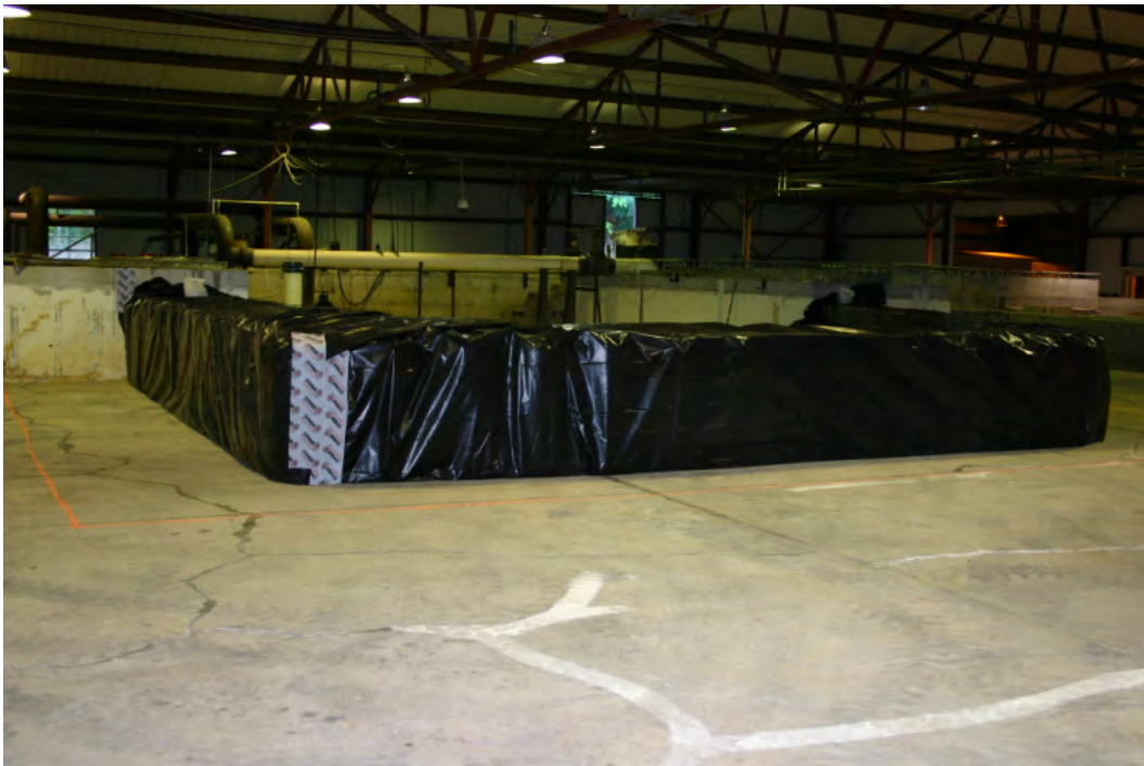
Figure 22. The finished barrier looking towards the 90 deg. bend in the layout.
