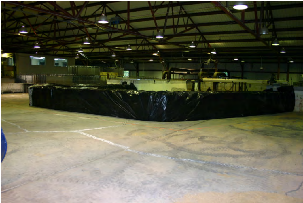
Figure 23. The finished barrier looking towards the 63 deg. bend in the layout.
