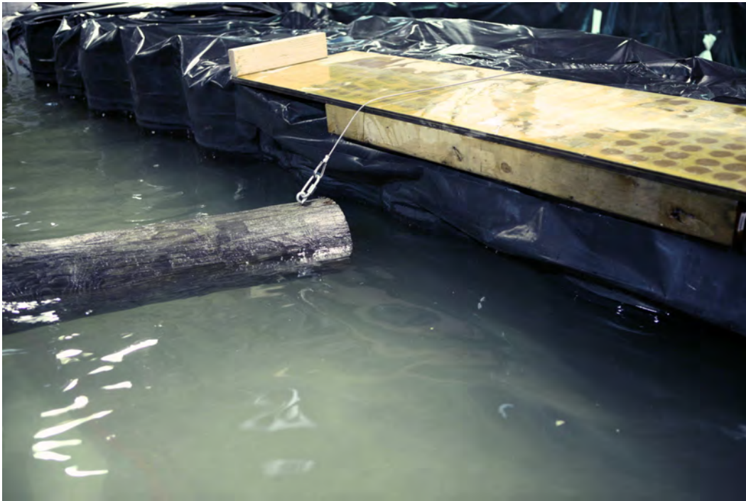
Figure 52. Log and protective plywood covering on the barrier.
