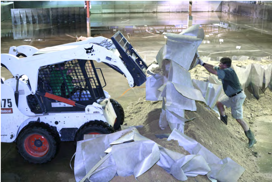
Figure 60. A forklift lifts the fabric from the top layer of Geocells.
