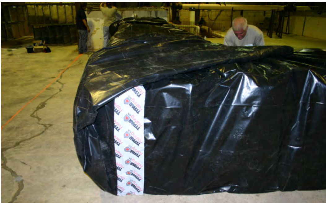
Figure 20. Flashing was used to tape the seams where two pieces of sheeting overlapped.
