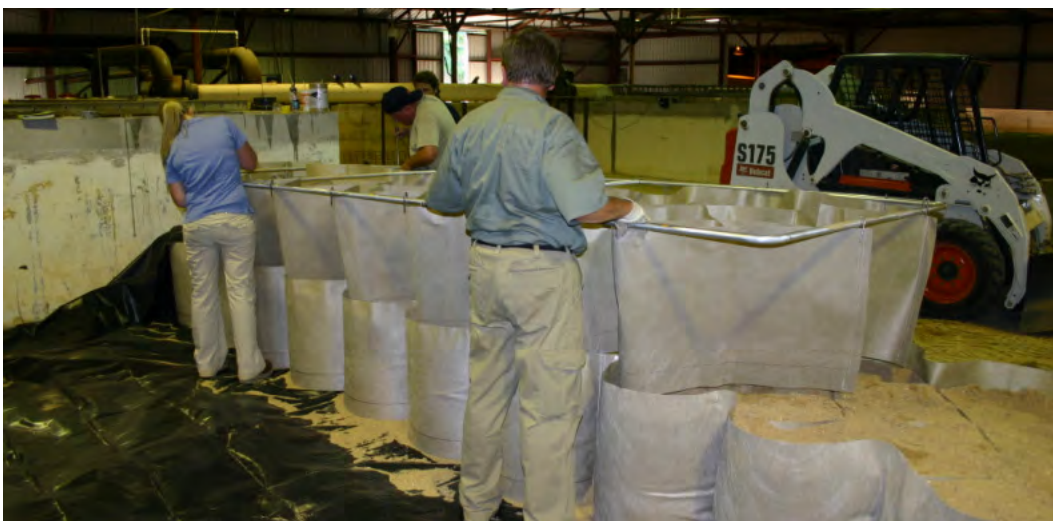
Figure 16. Starting the second layer of Geocells.
