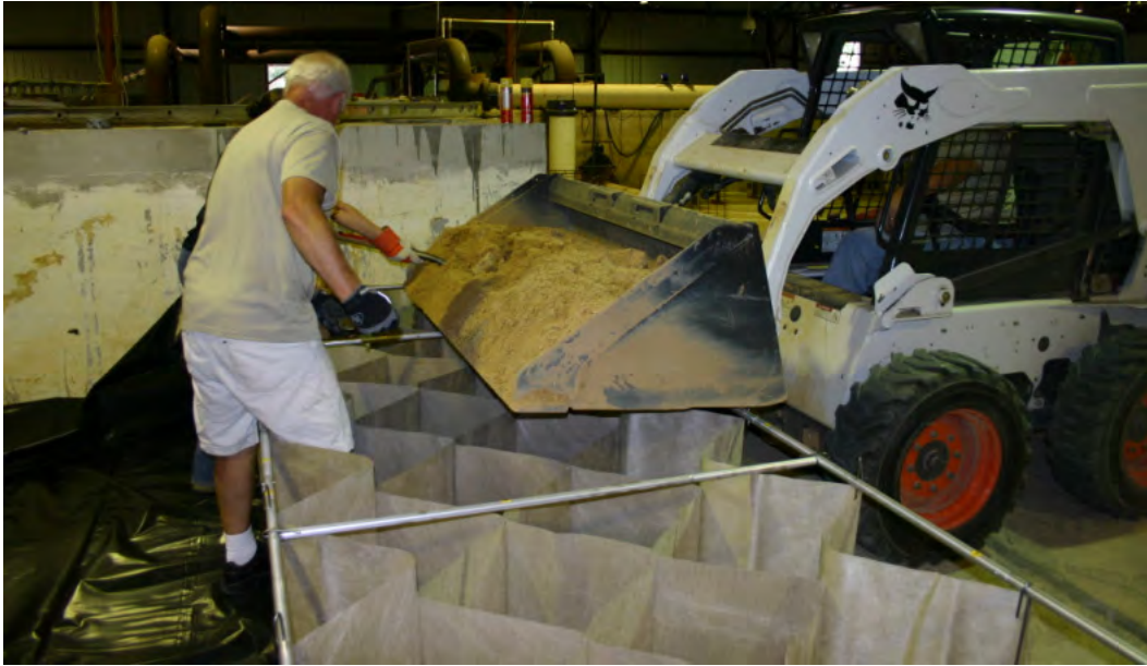
Figure 4. Typar® Geocell units being filled with sand.
