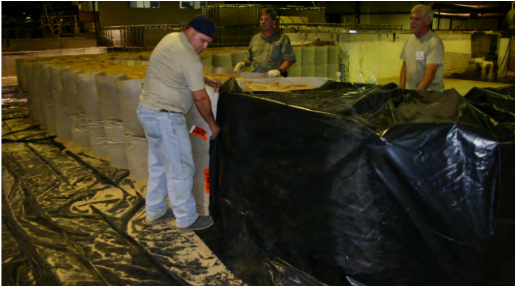
Figure 19. The plastic sheeting is being wrapped around the completed Geocell barrier.
