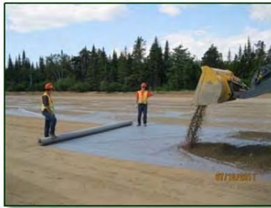
Unloading, spreading and levelling of the crushed stone.
