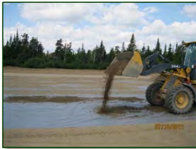
Unloading, spreading and levelling of the crushed stone.
