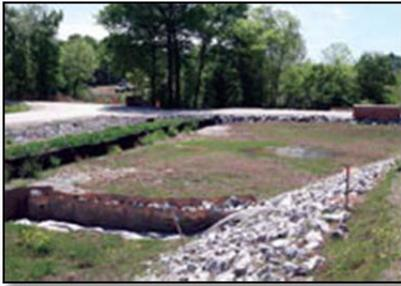
TYPAR Geocells (bottom), silt fences (left), rock check dams (right), and other best management practices can be used in combination.
