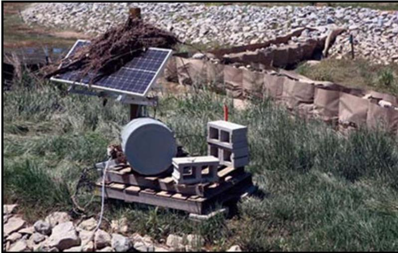
Debris on top of the solar panel indicates the high watermark from the 1,000-year rain event.
