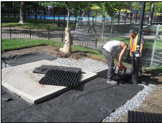
BodPave 85 installation over geotextile.
