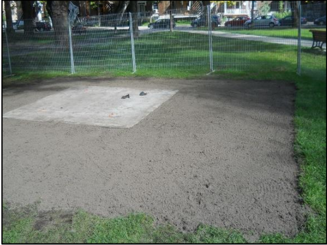
Covering BodPave 85 with stone dust.
