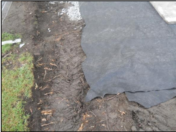
Geotextile application over stone ballast.
