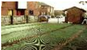
Mesh upon installation
