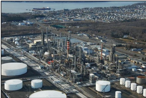
Ultramar refinery in Quebec City
