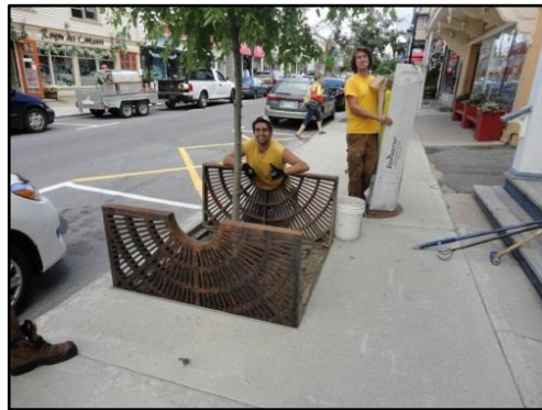
Removal of the metal grill
