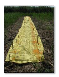
Mulch from the existing site was used to cover the Biobarrier membrane. Minimum cover is 2" and a maximum of 3".
