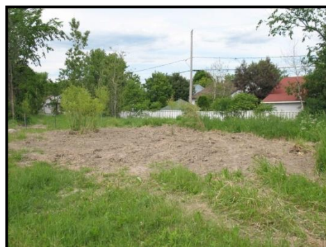
Soil was used to cover the Biobarrier membrane.
