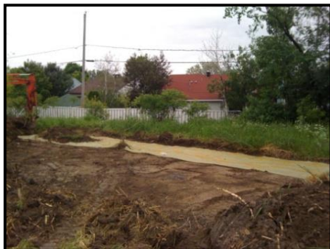
Placing the Biobarrier membrane.
